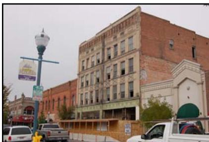
The Housing Company restored the Whitman Hotel in Pocatello. It now features 25 affordable apartments.
