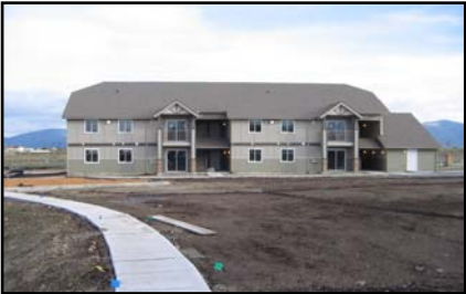
Tullamore Commons in Post Falls. This multifamily development was financed with tax credits.
