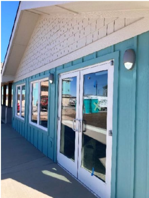
Clubhouse paint is completed.
